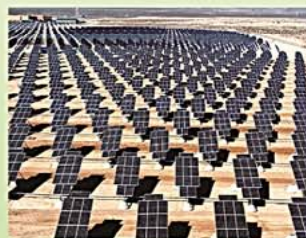
Solar Power Station
